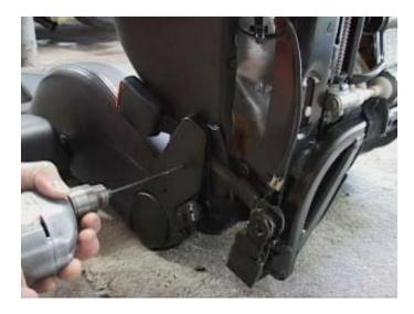
Time to separate the back and the bottom: just the two frames will be separated; the wires will remain connected.
