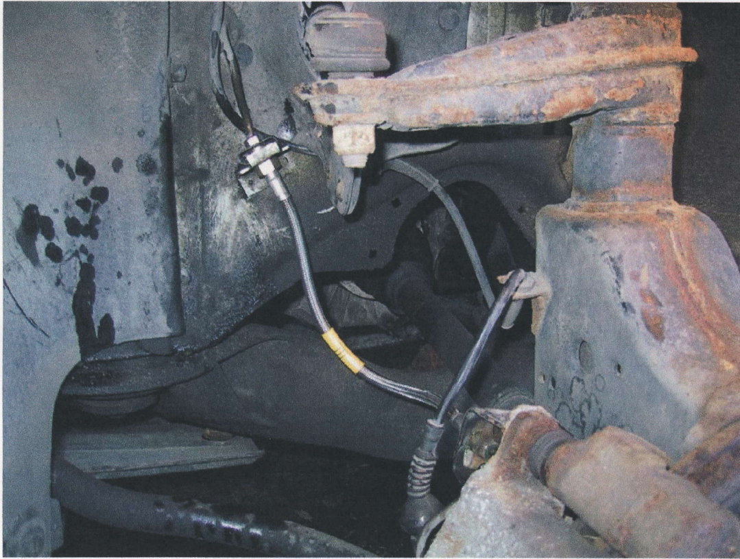
Photo 4 Installed Front SS line
